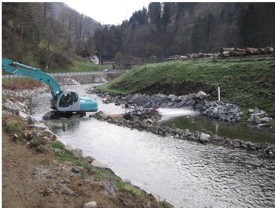
Slika 1: Gradbena dela na v.p. Ruta na Radoljni (foto: Rok Ferme) Figure 1: Construction work on the w.g.s. Ruta on the Radoljna River (photo: Rok Ferme)
