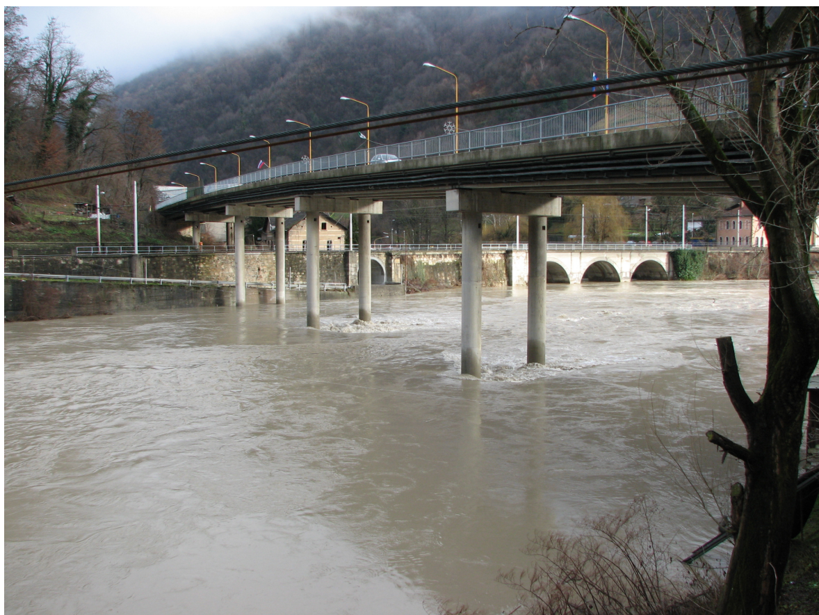
Visoka voda in povečana vsebnost suspendiranega materiala v Savi v Hrastniku, 26. 12. 2009 (foto: arhiv ARSO) High water and increased concentration of suspended material in the Sava River near Hrastnik, 26 December 2009 (photo: Agency Archives)
