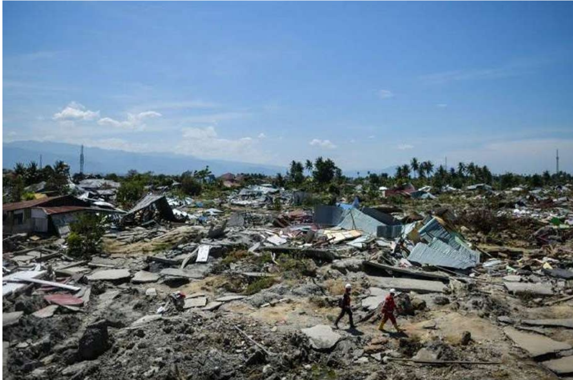
Slika 3. Uničeno naselje Perumnas Balaroa v Paluju (vir: https://news.abs-cbn.com/overseas/10/05/18/indonesia-survivor-recounts-doomsday-quake-horror ) Figure 3. Damaged Perumnas Balaroa village in Palu (Source: https://news.abs-cbn.com/overseas/10/05/18/indonesia-survivor-recounts-doomsday-quake-horror )
